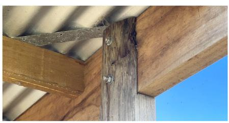
Poles with flat surfaces make for easy alignment and mounting of other timber.
